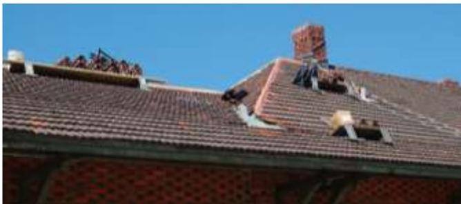
Portion of Railroad Museum tile roof showing tiles and wood ridge nailers. The brick pattern on the walls of the station is called “Flemish Bond.”
